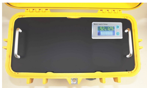
Battery Bank Inside View
